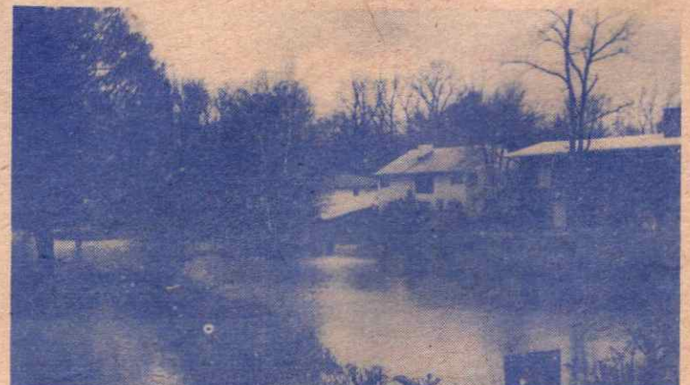
HIGH WATER, that's still with us, were the flood tragedies of 1972 and 73. The Thorofare Canal at the north end of the island looked like this in those days.
